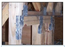
Connector at the End of the Wall Unless otherwise noted, bending steel in the field may cause fractures at the bend line. Fractured steel may not carry load and must be replaced.
