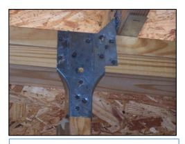
Connector Overlap Options to make this work include using a different connector, like twist straps or installing a hurricane tie on the other side instead of on the left.
