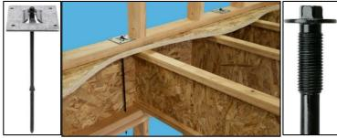
Stud-to-plate connections are required to complete the load path.
